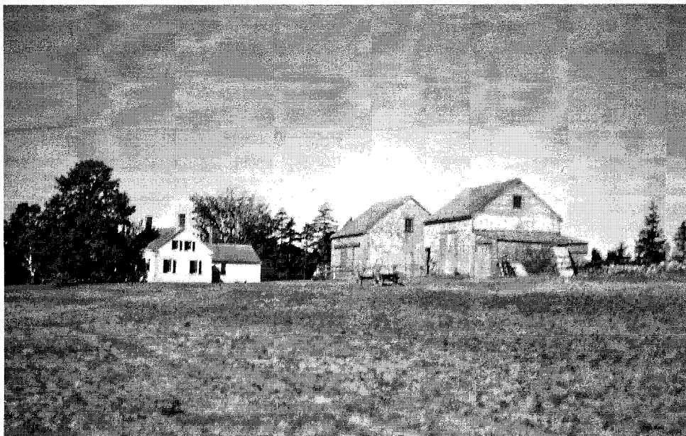
The Stephen Orr farm. Stephen Orr was a rock slooper as well as a farmer. At least one of these barns had been built in 1850. Note that the door is NOT in the gable end. This is the older style known as an English barn. (Formerly Higgins now Dayton's)
