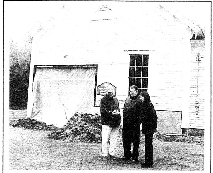
Architect Carol Wilson, President Phil Jordan, and Kenneth Hamilton discuss brick replacement in front of schoolhouse
