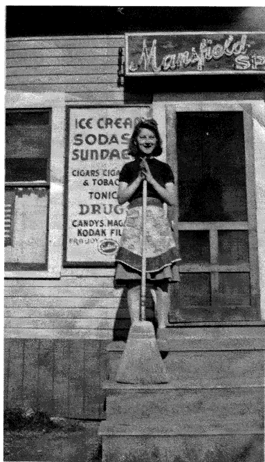
Charlotte Stilphen on the job at Bert's
